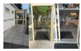
Ramp width = 180cm, external door width = 104cm, internal door width = 98cm
